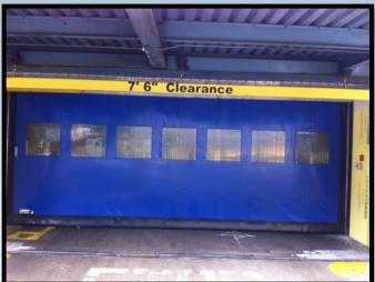
Thanks to reports filed through the SMS Confidential Hazard Reporting System, the Airport found a substitute for the strip curtains (plastic meat locker-looking strips) to keep the Terminal 1 Baggage Make-Up Area warm and the water pipes and fire lines flowing. That alternative: zoom doors.
