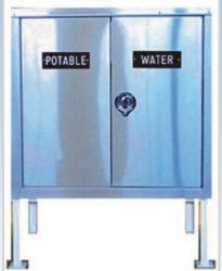
There are approximately 40 Potable Water Cabinets, mounted in a variety of ways and locations throughout the Airline Ramp. These Cabinets expedite the dispensing of potable water, better known as drinking water, directly to aircraft parked in congested loading locations. It is important to remember to close the Cabinet when not in use.
